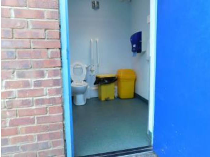
Disabled toilet exterior
